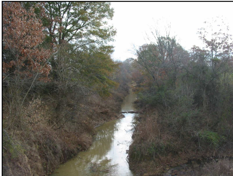
Figure 1. Johnson Creek near Hernando
