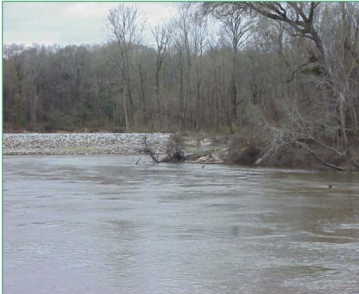
Walkiah Bluff Diversion Structure
