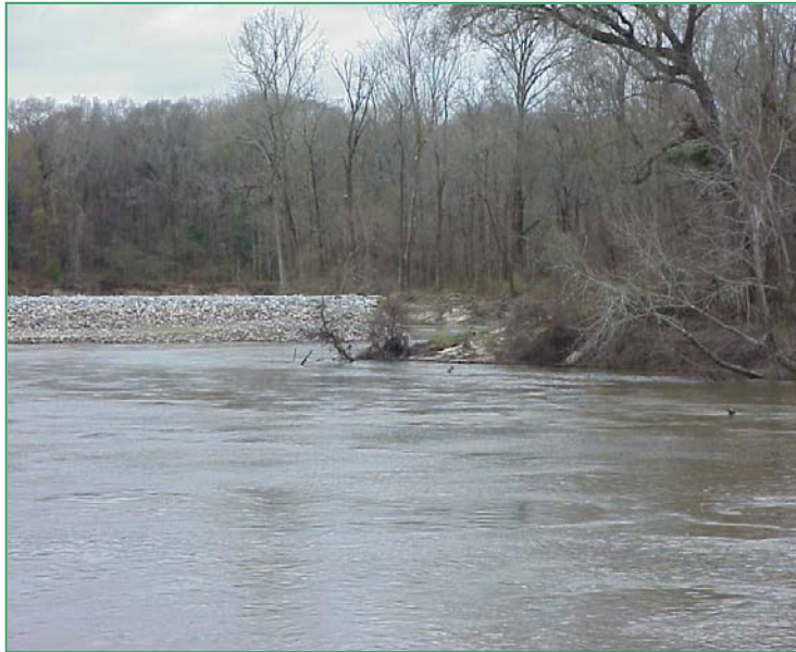
Walkiah Bluff Diversion Structure
