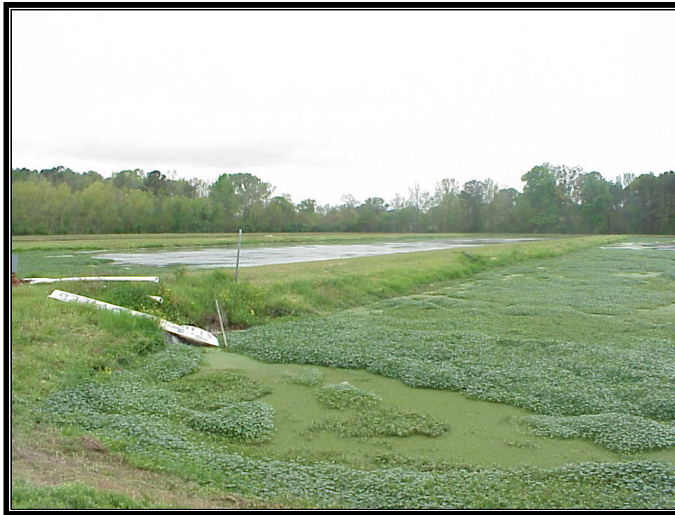
Photo 2. Newton POTW Facility, Aquatic Weed Coverage in Cell 3
