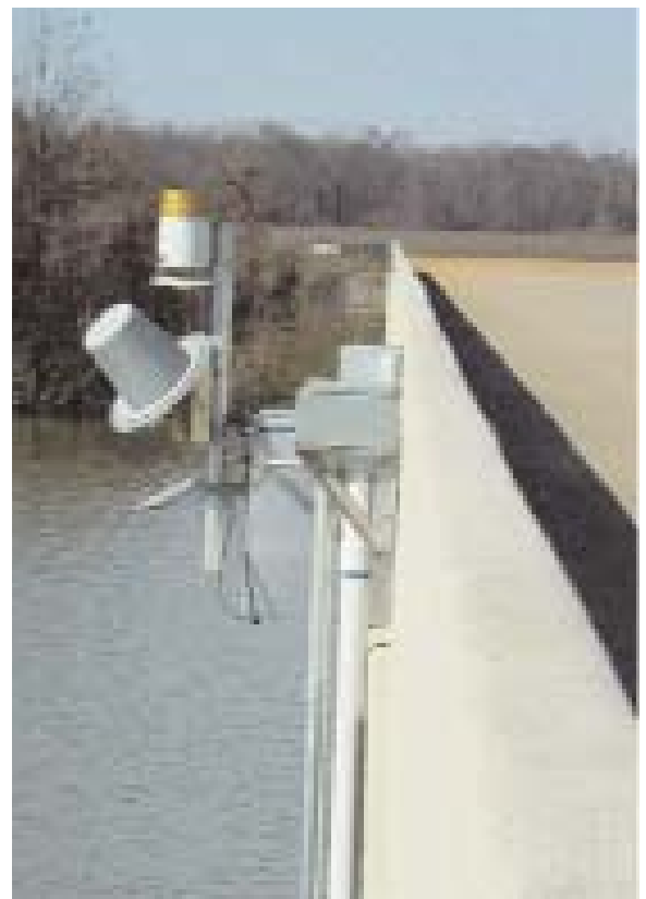
USGS Monitoring Station installed on Bee Lake in the fall of 2005.
