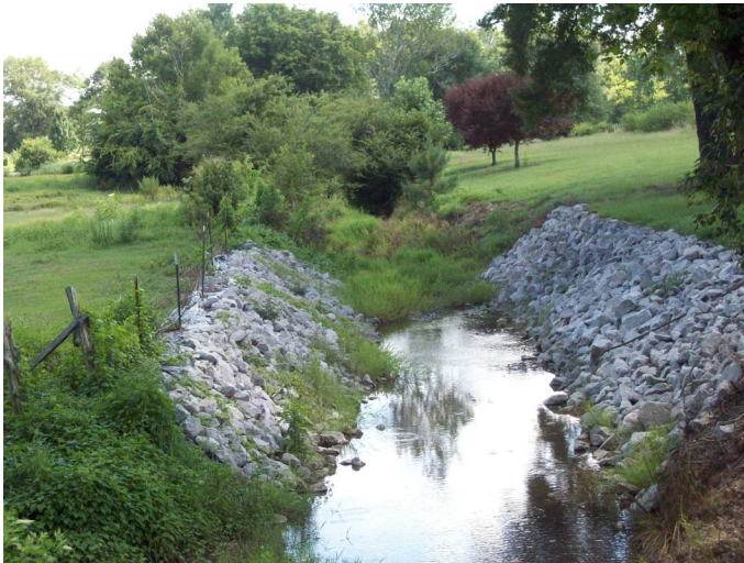
Photo 3 – Previously stabilized stream bank, Golden, MS
