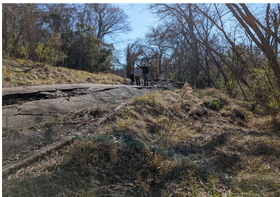
Slope failure in Pleistocene loess disrupting road infrastructure on Union Avenue in Vicksburg National Military Park highlighting the constant threat of geohazards posed by the thick loess cover throughout the geologic mapping project area. Photo taken in Section 9, Township 16 North, Range 4 East.
