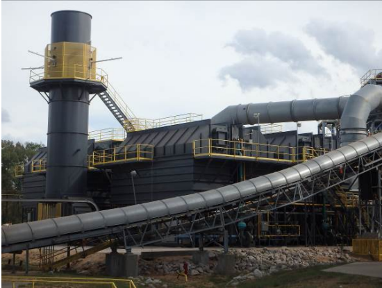
19) Regenerative Catalytic Oxidizer and Burner
