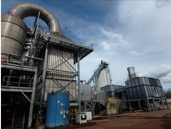
7) Wet Electrostatic Precipitator and Regenerative Thermal Oxidizer
