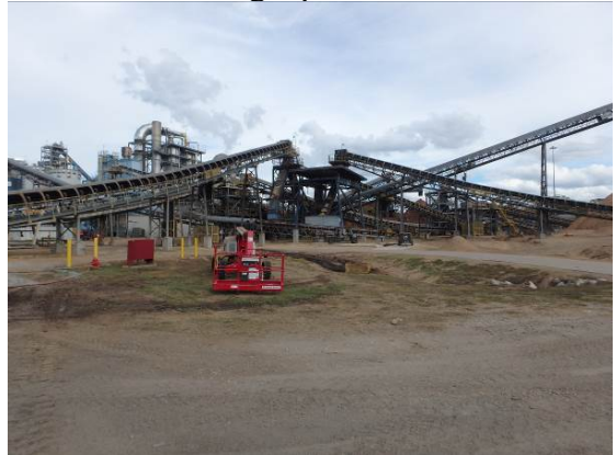
5) Green & Dry Wood Transfer/Handling Ops
