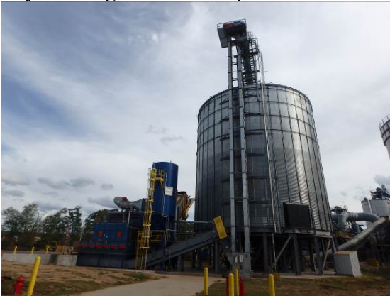
20) Dry Shavings Truck Dump
