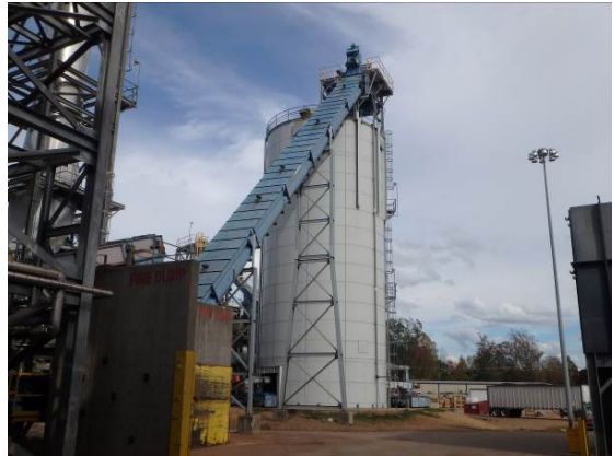
11) Hammermill Feed Silo w/ Bin Vent
