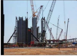
Combined cycle facility under construction, slated to begin commercial operations in 2018
