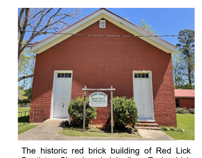
The historic red brick building of Red Lick Baptist Church (originally Red Lick Presbyterian Church), built from locally crafted brick in 1846. Section 55 Township 10N, Range 2E. Photographed on March 8, 2022.
