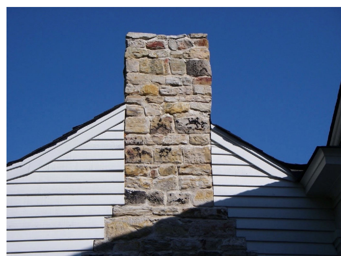
Catahoula sandstone chimney of the Porter House built around 1830 and moved to Raymond, Mississippi, in 2004. Photographed on September 20, 2004.
