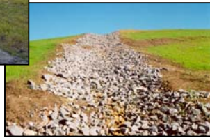
Grouted Rip Rap
