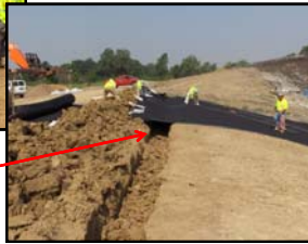
Roll liner onto prepared surface
