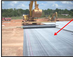
Spreading soil over GCL with low-ground pressure equipment
