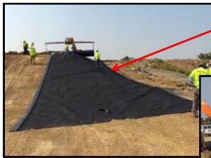
Place liner in anchor trench at top of slope
