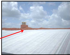
Rolling out GCL on prepared surface
