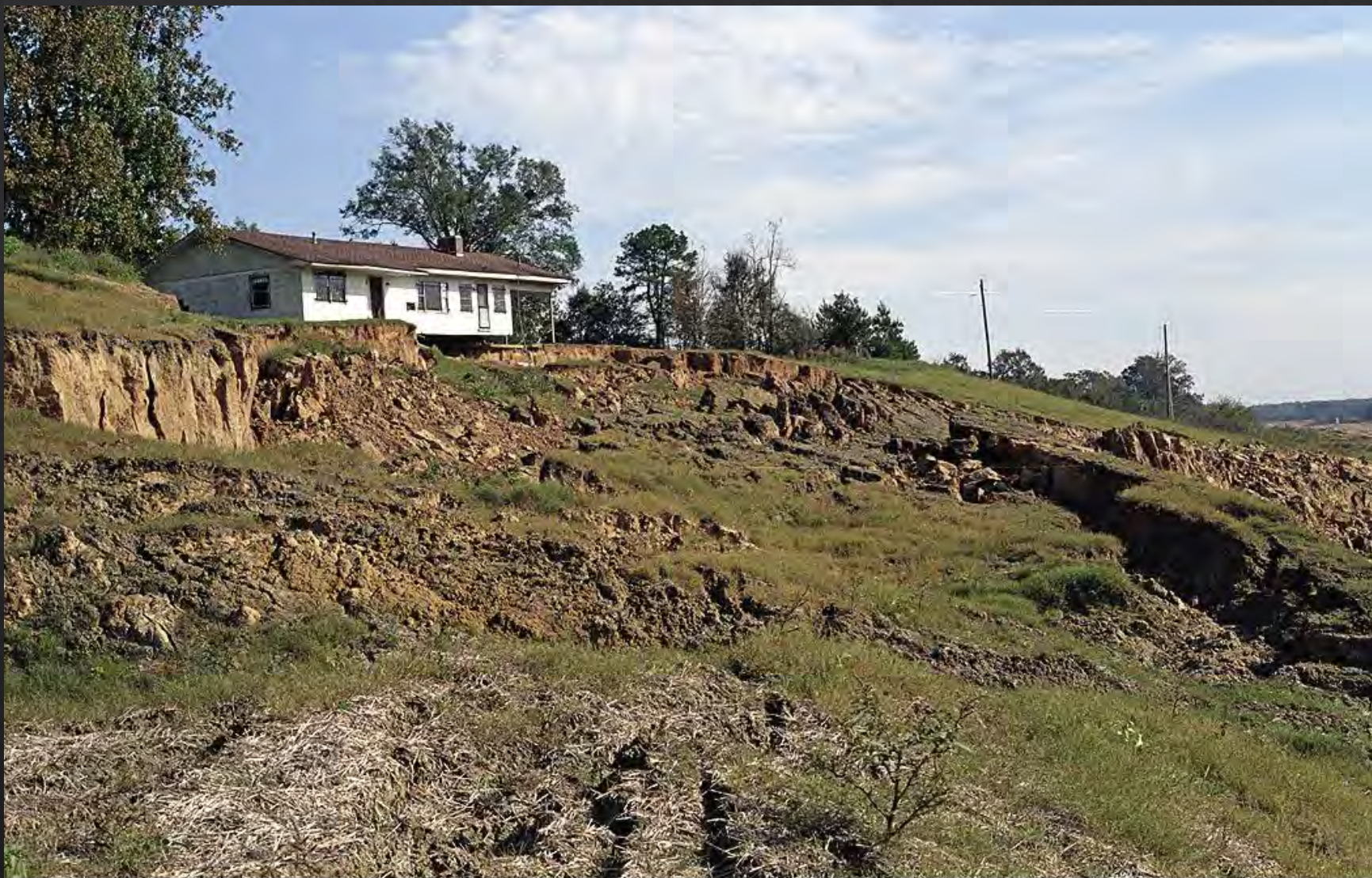
Figure 1035. Slump in loess and underlying Miocene clays cutting into the foundation of the Keating house on Highway 61 at Cannonsburg in Jefferson County. The slump occurred when the toe of the hill was cut to expand the highway. Picture (color negative 536-20; Image 334) taken on November 16, 2004.
