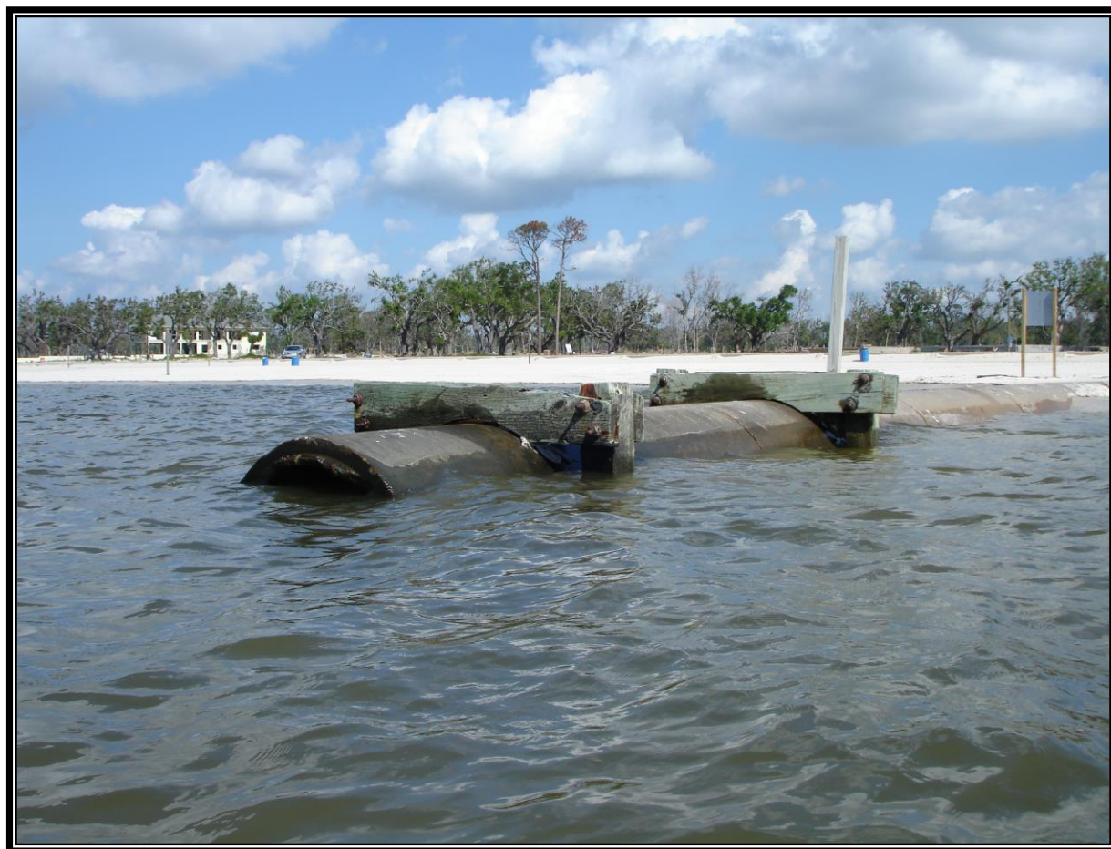
Figure 35. Typical Storm water Culvert discharging on the Beach
