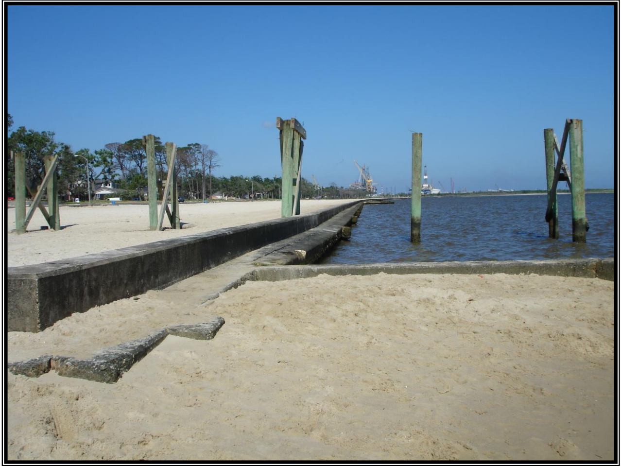
Figure 34. Concrete Seawall at Pascagoula Beach and Remnants of Pier destroyed by Hurricane Katrina
