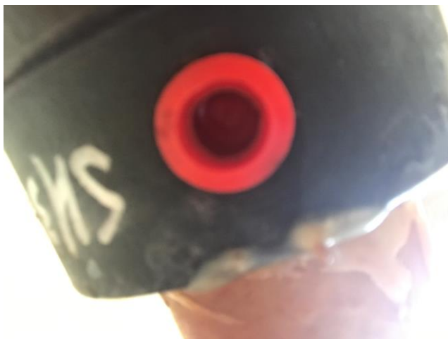
Same penetration fitting. Factory plug not removed.
