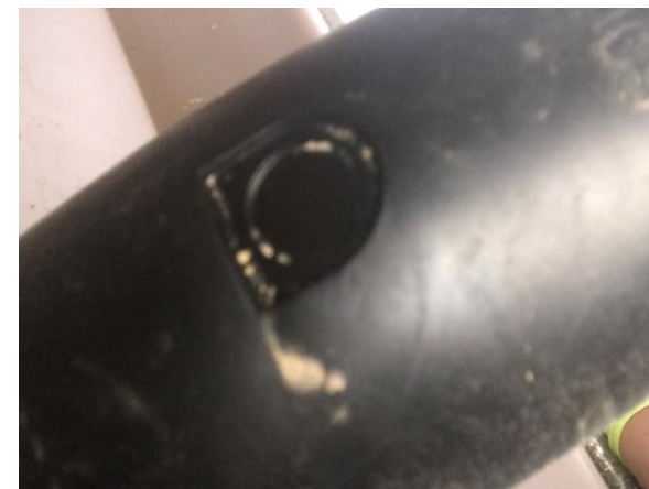
UPP fitting. Appears open right? It's not. Clear plastic covering it.
