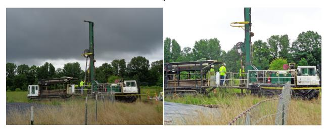
Figure 4. Sonic drilling rig coring at the Southeastern Wood Preserving Superfund Site on June 19, 2017, in stormy and fair weather.
