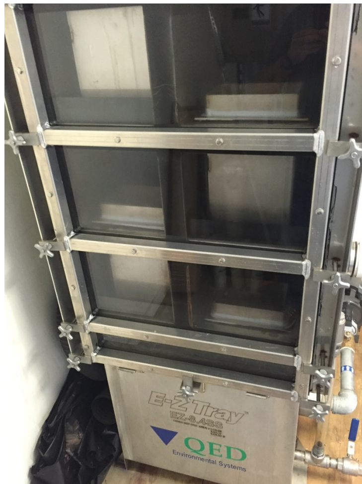
Picture 3 – A typical Compact Tray Air Stripper System
