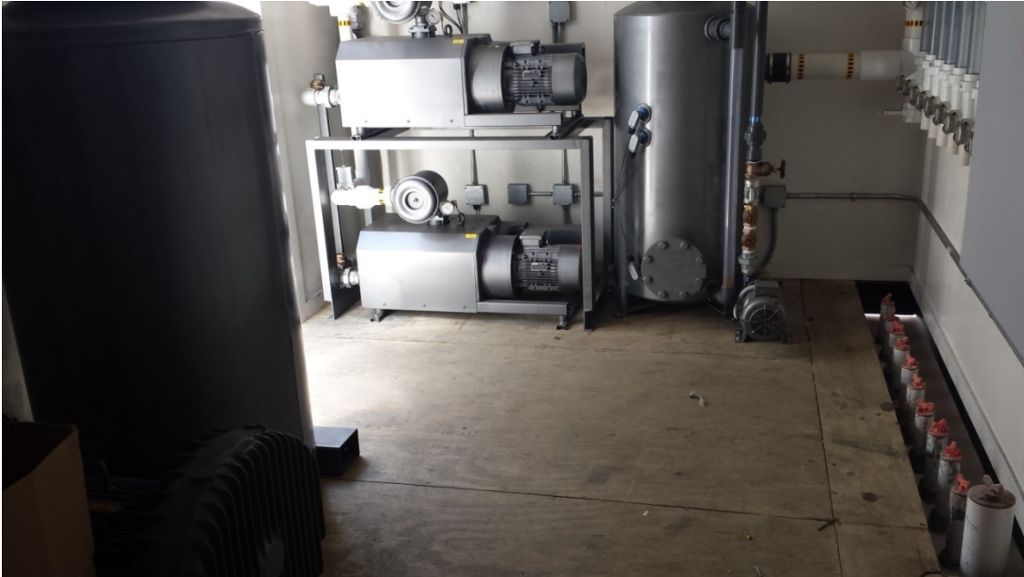
Picture 1 – Typical High Vacuum Dual Phase Extraction System Blowers and VLS Vessel Connection
