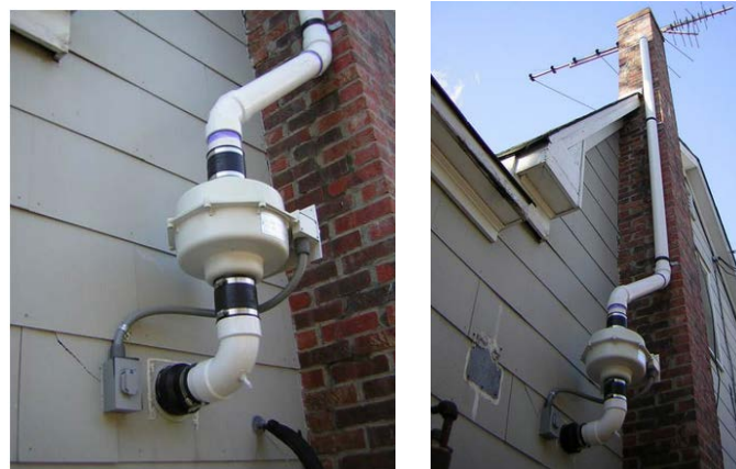
An example of stack piping equipped with an electrical fan
