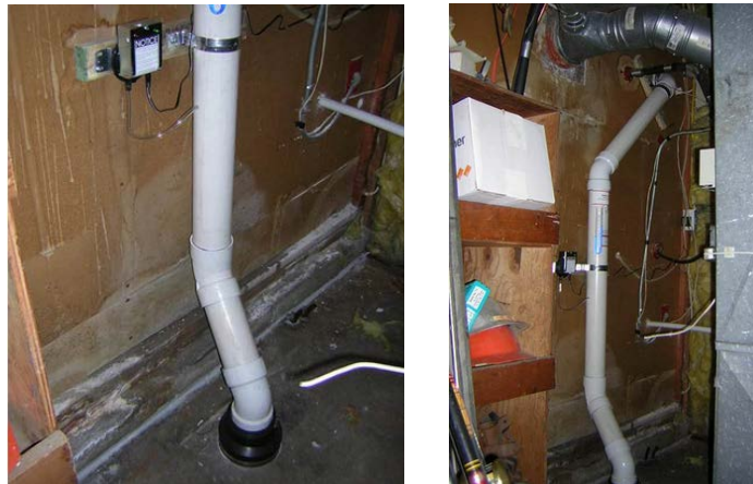
An example of extraction point and exhaust piping equipped with a negative pressure manometer
