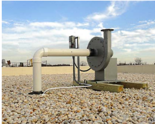
An example of large radial blower application
