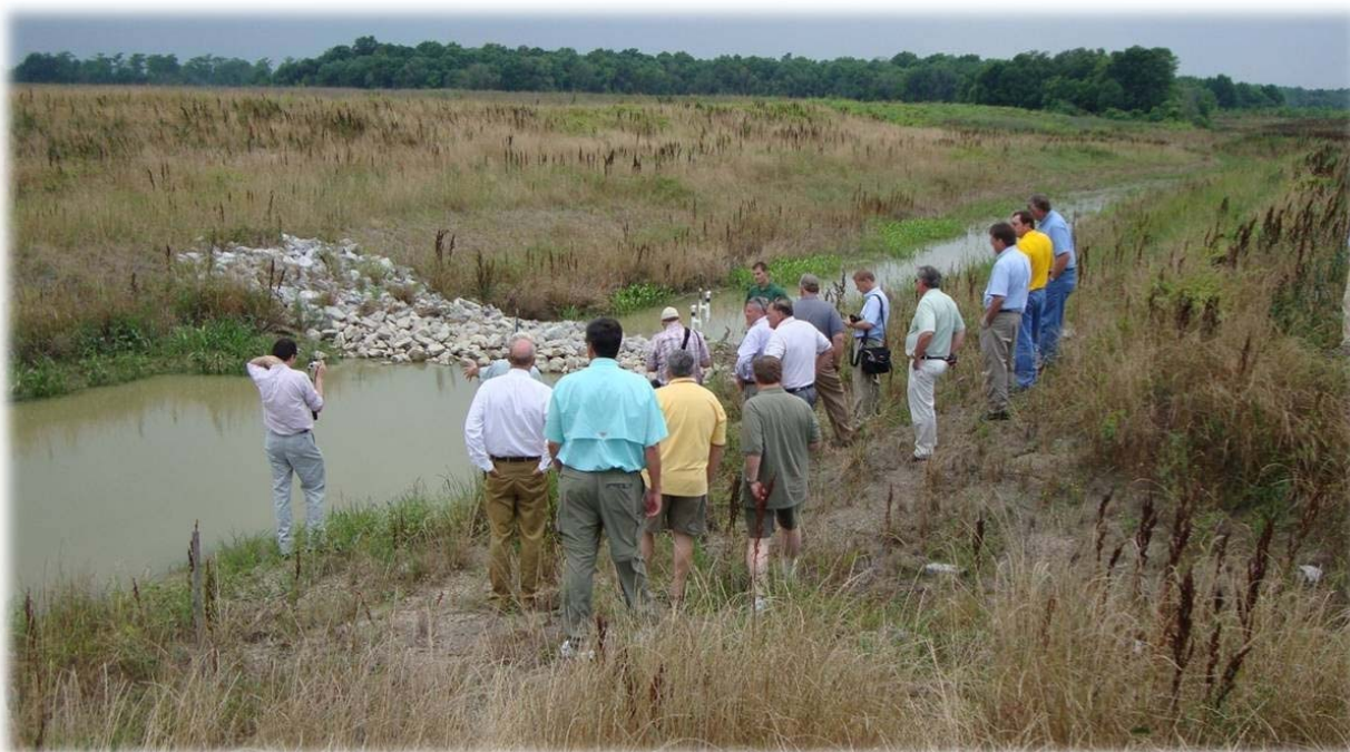
Figure 12. Low head weir implemented in the Delta for sediment retention and denitrification.
