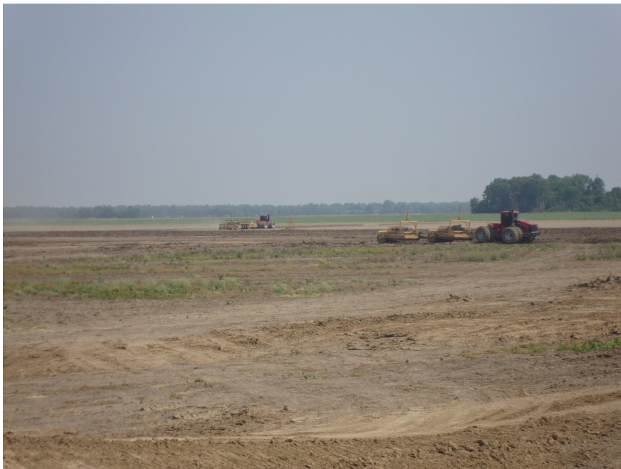
Figure 11. Land leveling to improve irrigation efficiency in the Delta.
