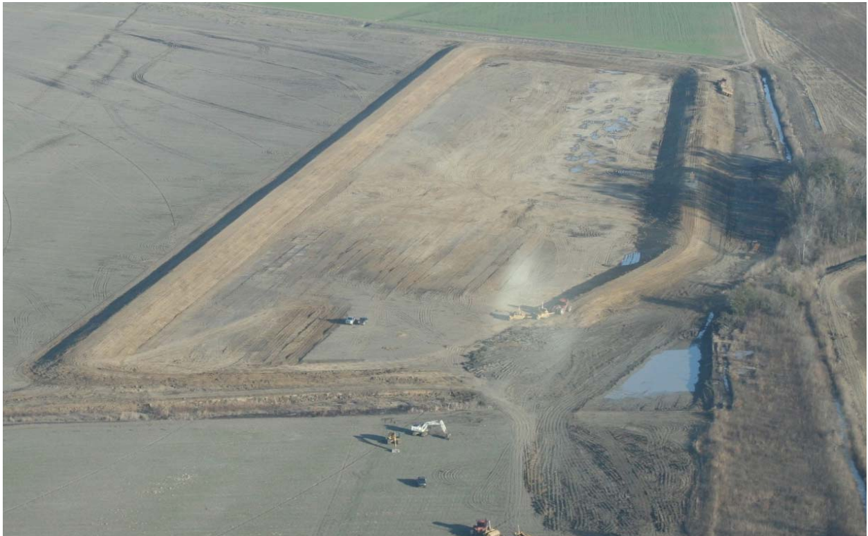
Figure 9. Aerial View of on-farm storage reservoir being constructed in the Delta.
