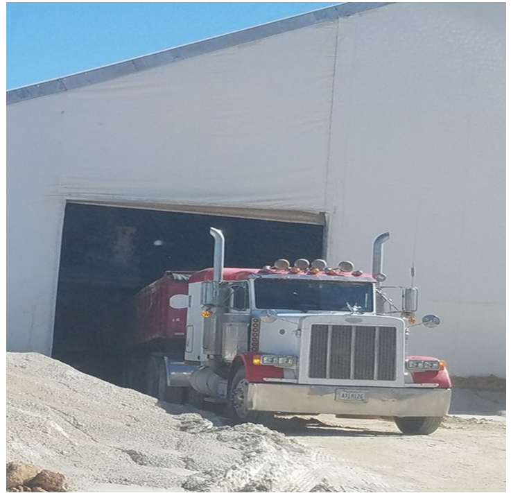
Figure 4. Tank ET-10 Sludge Removal Project: Loading dump truck within the temporary structure over the IB with solidified ET-10 material. The dump truck was used to transport the material off-site for disposal.
