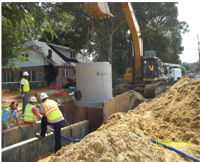
Figure 6. Providence Street Sewer Line Replacement Project. Contractor replacing a manhole along Providence Street.
