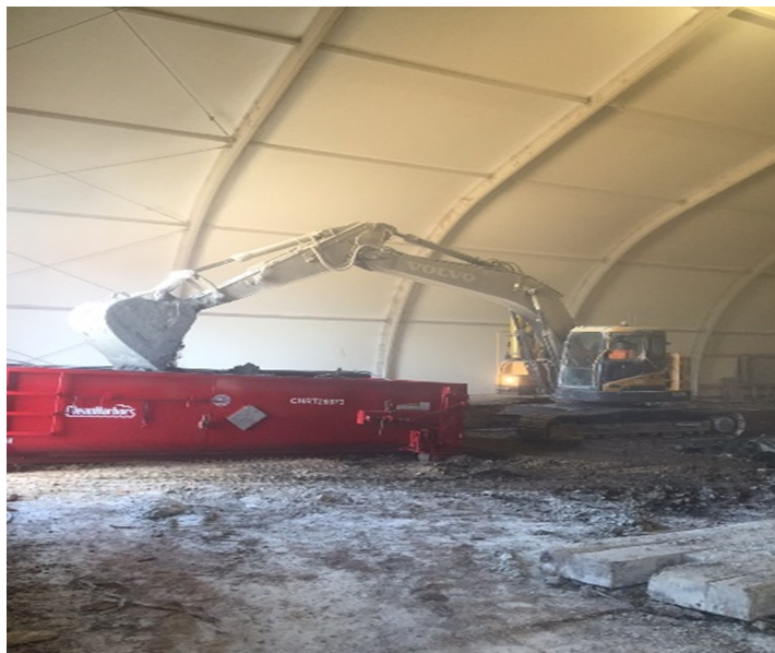
Figure 8. Structure Dismantling Project. Contractor demolishing an on-site warehouse and preparing the material for recycling.
