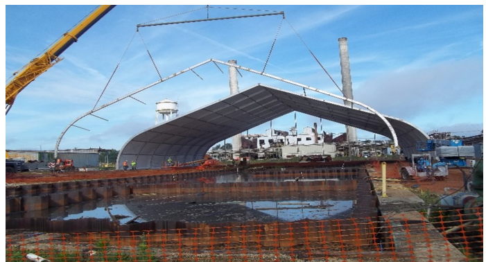
Figure 1. IB Decommissioning Project. Contractor installing temporary structure over the IB.
