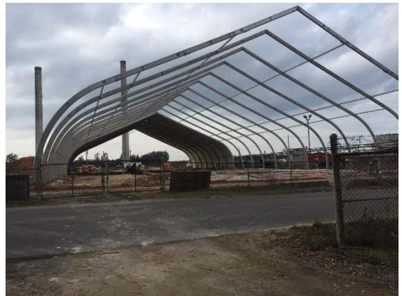
IB tent structure demobilization progress
