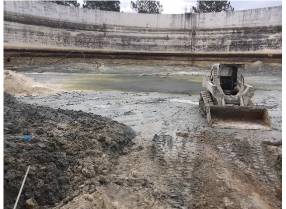
Stabilization of material within ET-10
