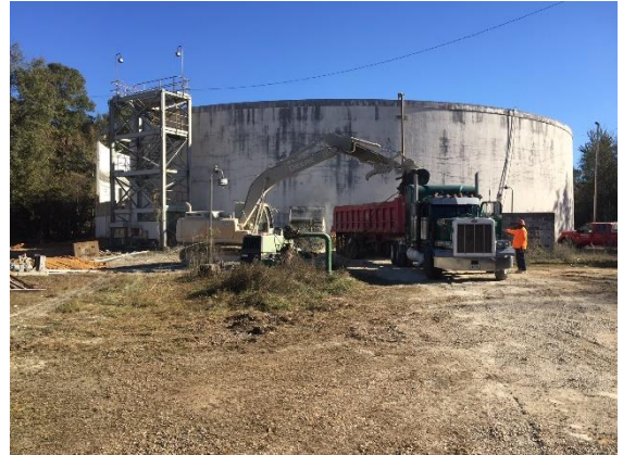
Material loading at ET-10
