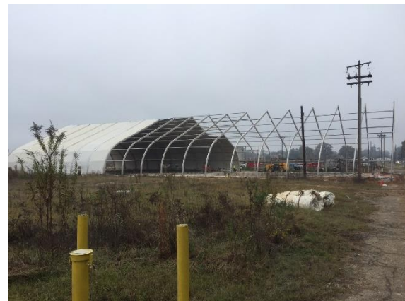
IB tent structure demobilization progress
