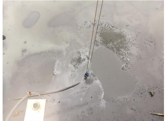
Transfer pump located inside ET-10
