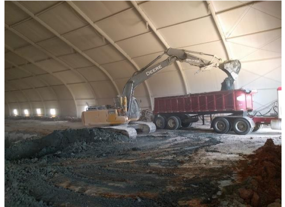
Stabilized Batch #3 material loading out for disposal
