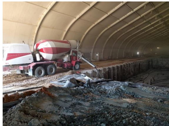
Flowable fill placement in Cells #1 and #3
