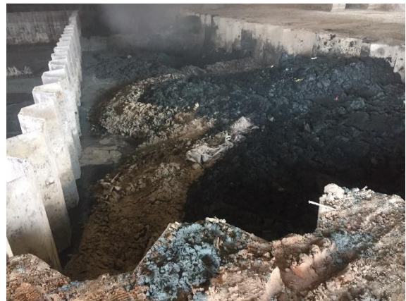
Stacked material within the IB
