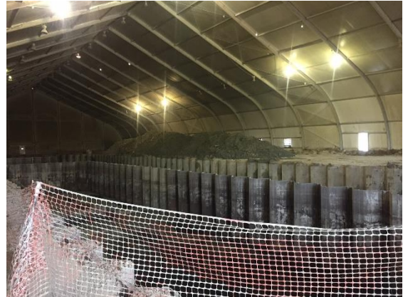
Batch #2 material stacked on the side of the IB
