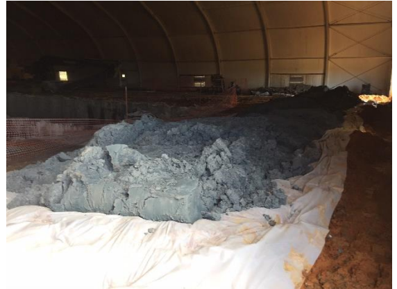
Batch #1 material stacked on the edge of the IB
