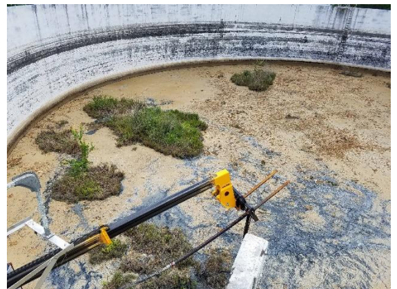
Pumping operation inside ET-10
