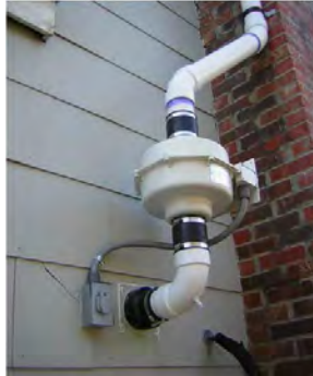
An example of stack piping equipped with an electrical fan
