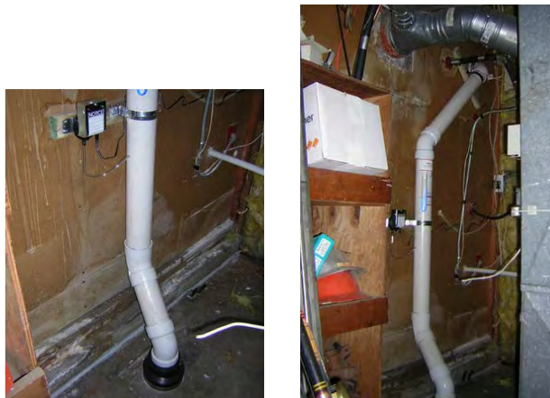
An example of extraction point and exhaust piping equipped with a negative pressure manometer
