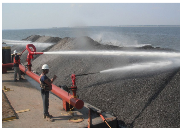
Using a pump and nozzle system, crushed limestone was deployed from a spray barge to enhance existing Mississippi oyster reefs.
