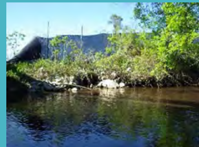
Stormwater outfall into Turkey Creek
