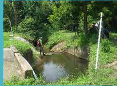
Bank erosion and streambed sedimentation
