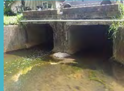
Railroad bridges and pipes
