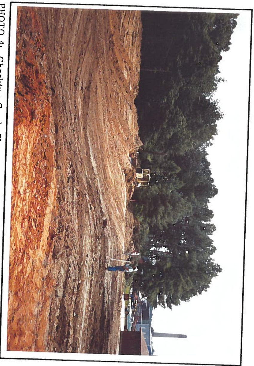
PHOTO 3: Cut and Fill of Dike Material Using D5H and D6H Dozers
