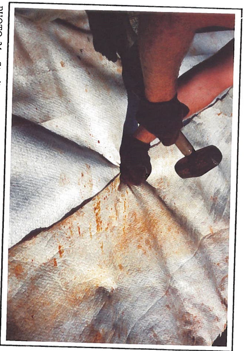
PHOTO 23: Folding Back Filter Fabric on West Side
