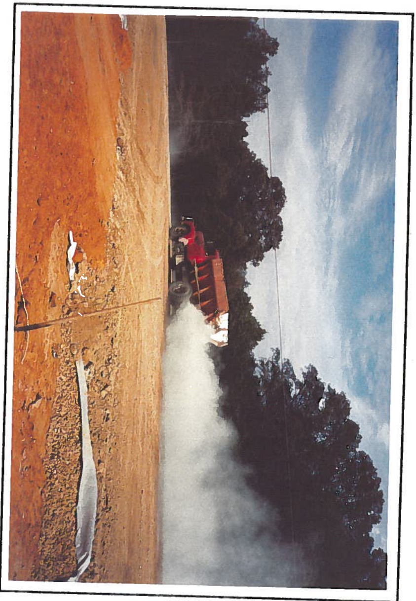
PHOTO 27: Applying Limestone with Truck-Mounted Agricultural Spreader
