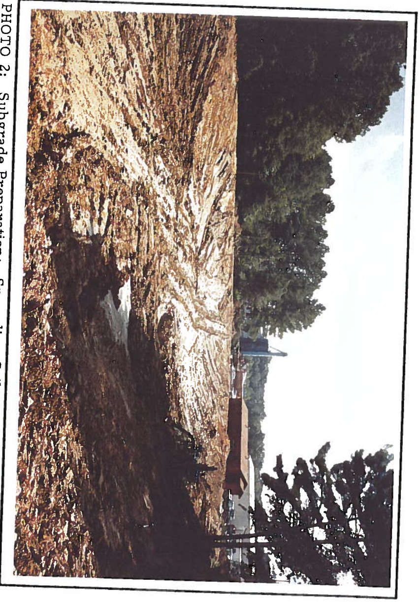
PHOTO 1: Subgrade Preparation: Dewatering and Tracking
