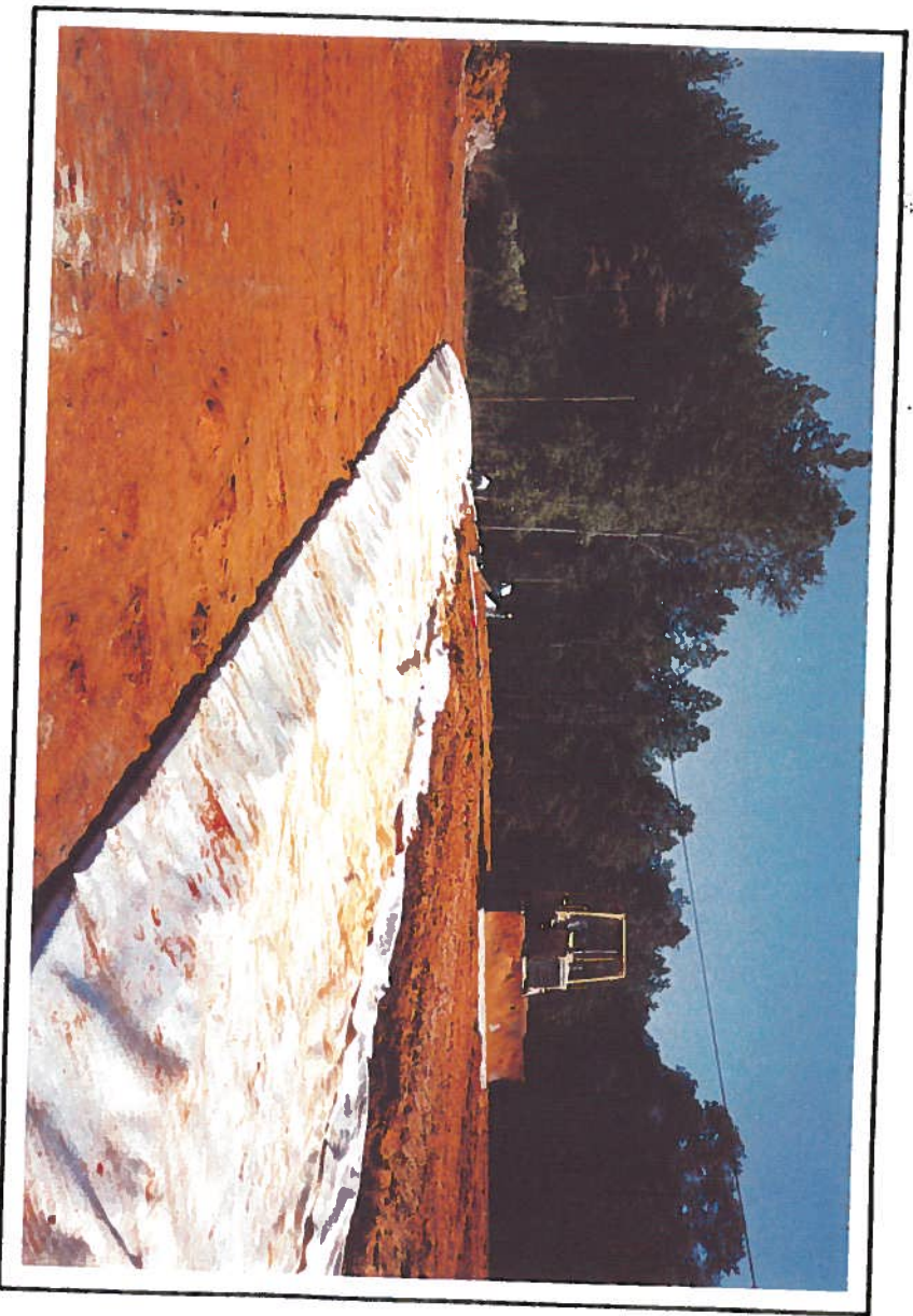
PHOTO 23: Folding Back Filter Fabric on West Side
