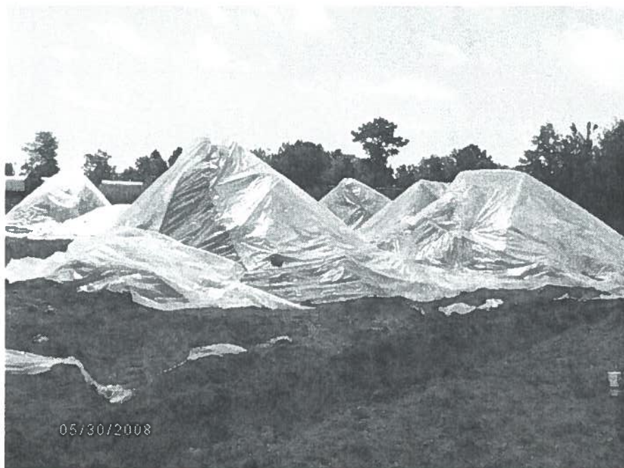
Representative photo of covered soil stockpiles
