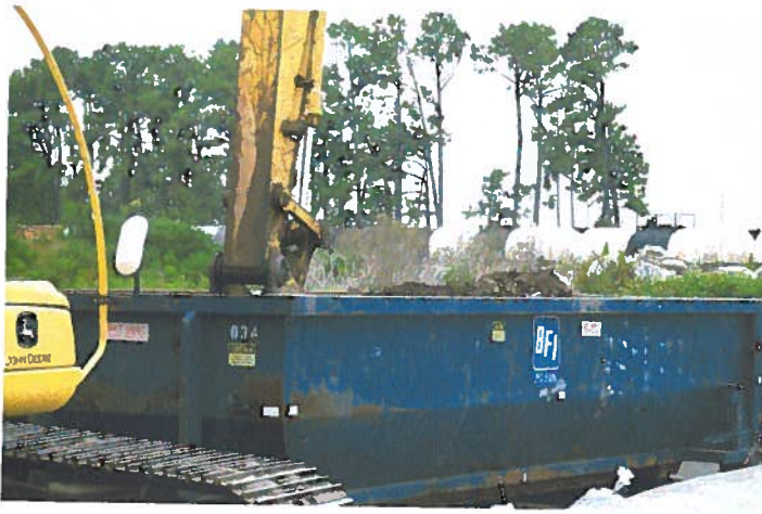
Mixing 10 yds soil with amendment material
