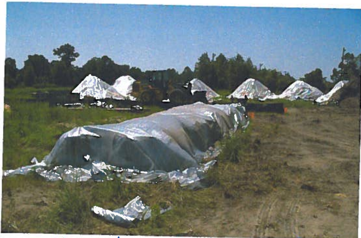
Background - Stock piles of soil to be treated Foreground - amendment material to dust soil
