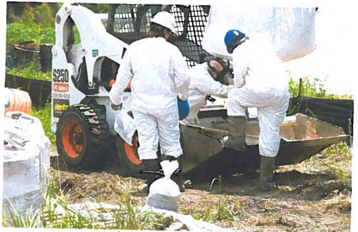
Measuring treatment material into Bobcat bucket
