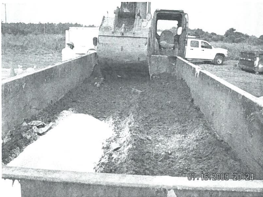
Soil treatment mixing container. Soil and treatment amendment material.
