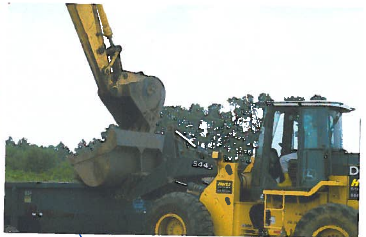
Finished mixing - moving to loader for transfer to storage area
