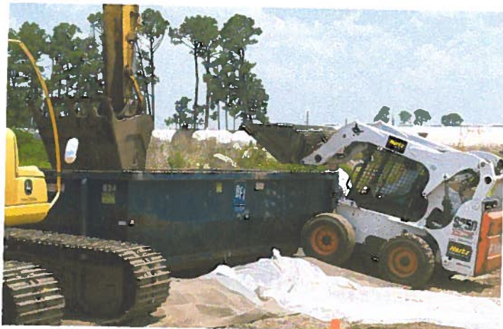
Bobcat - transferring treatment material to treatment containers
