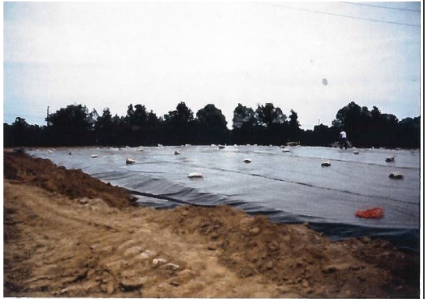
Installation of plastic cap during closure of the Equalization Lagoon in 1993
