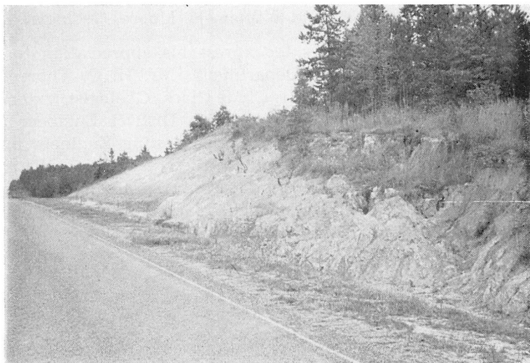
Figure 15.—Zilpha clay slide in southeast cut of highway at mile 57.0. September 13, 1962.
