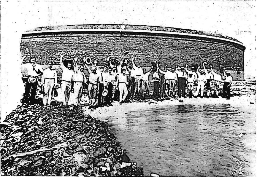
Figure 12.—An illustration of historic beach erosion. Photo was taken in 1926 when a narrow beach still existed on the Sound side of Old Fort Massachusetts, Ship Island. Today the Fort is nearly surrounded by water as the Sound shore has receded and the Gulf side advanced seaward. Photo compliments of Mr. J. R. Anderson, Gulfport, Mississippi.
