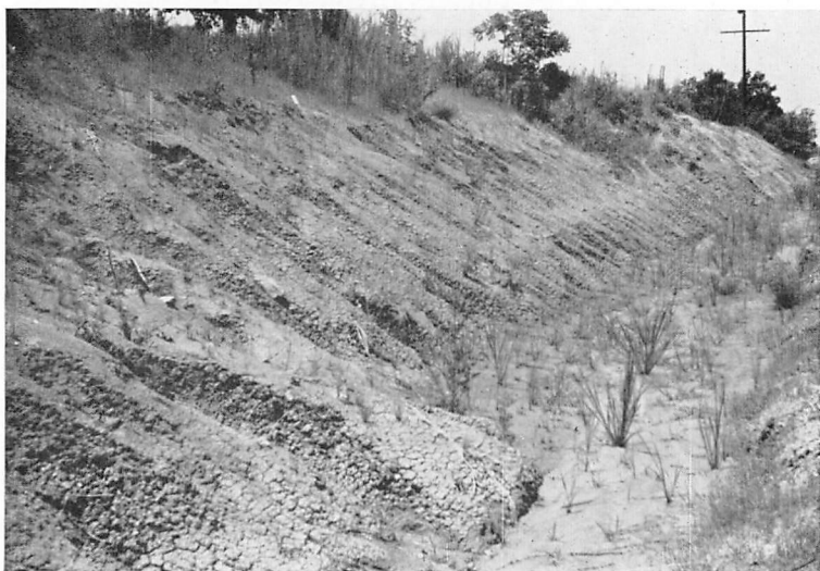
Figure 5.—Weathering Porters Creek clay exposed in a cut (NW.¼, SE.¼, Sec.24, T.12 S., R.1 E.) of a road on the lower south slope of the Skuna River valley 2.9 miles east-northeast of State Highway 341. July 21, 1961.
