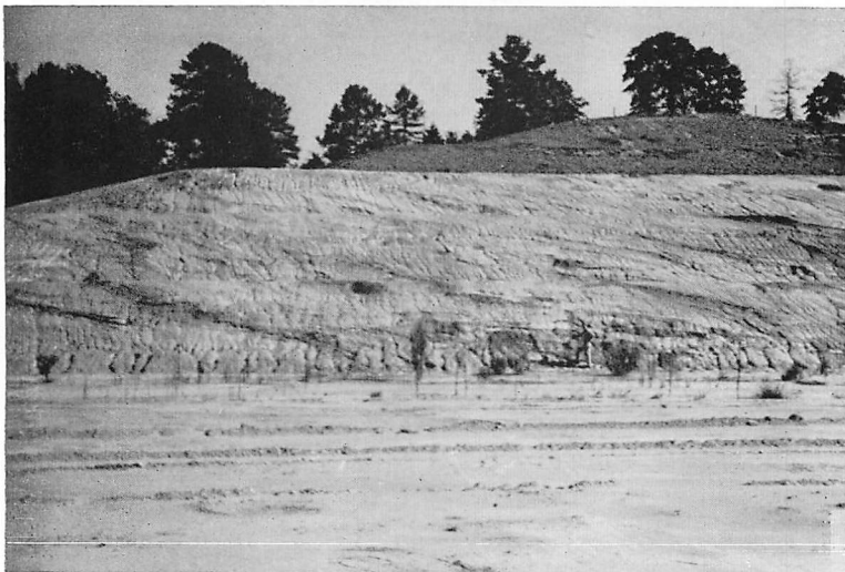
Figure 8.—Zone 5 Wilcox (Hatchetigbee) complexly intertongued and inter-lensed silts and clays (light) overlain by terrace sand (dark) in south cut of Interstate Highway 20 just east of Meridian, mileage 15.6. September 4, 1960.
