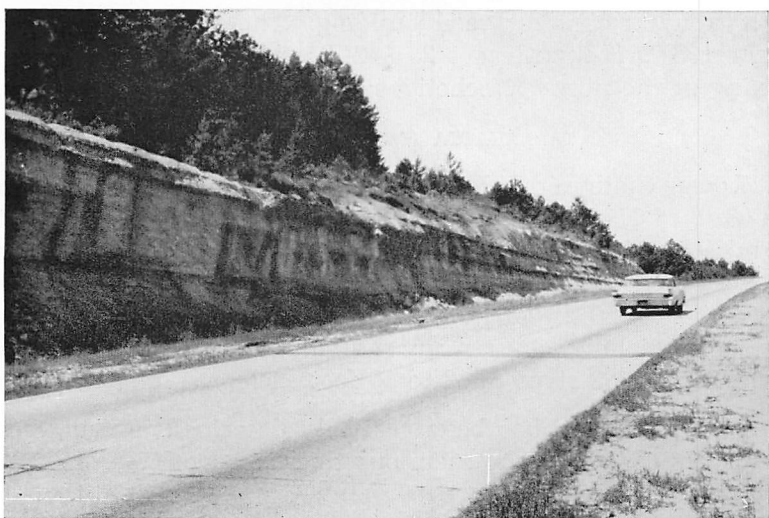
Figure 13.—Upper Tallahatta thin-bedded siltstones overlain by weathered Winona greensand, top of south cut, U. S. Highway 80, mileage 29.9, 9 miles west of Meridian. September 4, 1960.
