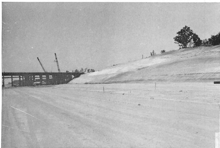
Figure 6.—Intertongued Bashi zone silty sands and silty shales. Light beds at left are buff-colored silty sands. Dark beds at right are silty shales. North cut at underpass south of Russel, Interstate Highway 20, mileage 12.2. September 4, 1960.
