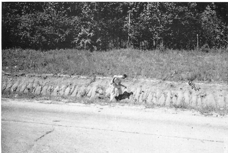
Figure 16.—Badly weathered Archusa-Potterchitto marls, north cut, U. S. Highway 80, one mile east of Newton at mileage 44.8. September 4, 1960.
