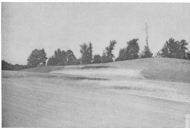
Figure 7.—Intertongued Bashi zone lignites (dark), carbonaceous silty clays (lighter), and blocky clays (very light). North cut, Interstate Highway 20, mileage 8.5. September 4, 1960.
