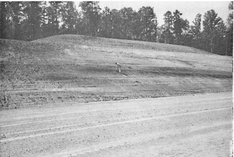
Figure 4.—Zone 3 Wilcox thin-bedded silty clays (light) and lignite (dark), south cut, new Interstate Highway 20, mileage 7.4, one mile west-southwest of Toomsaba. Strata dip noticeably west. September 4, 1960.
