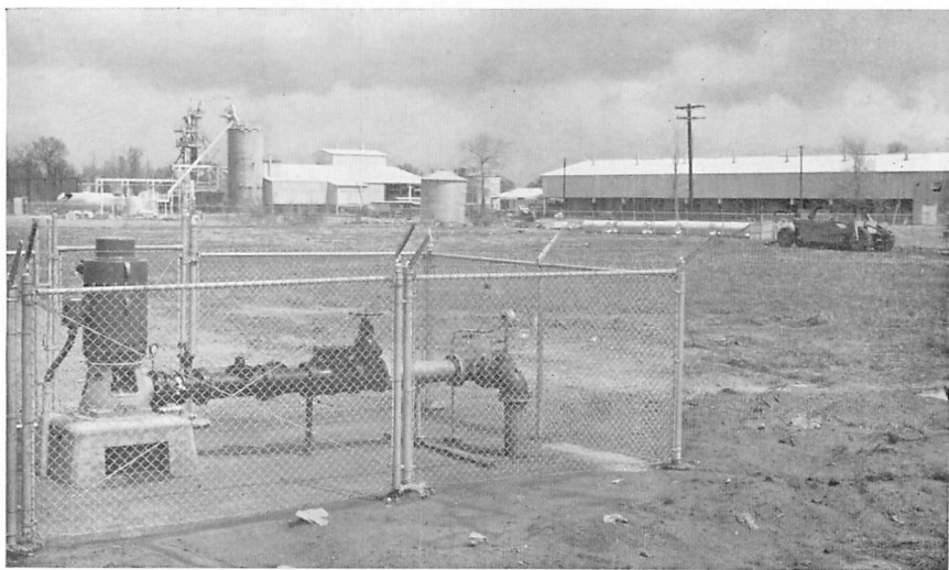
Figure 4.—Well in the Gordo formation in Monroe County. Four such wells averaging about 415 feet deep furnish the water supply for plant in background. Wells flowed 500 gpm or more each when installed, and are pumped at rate of about 1,000 gpm each.
