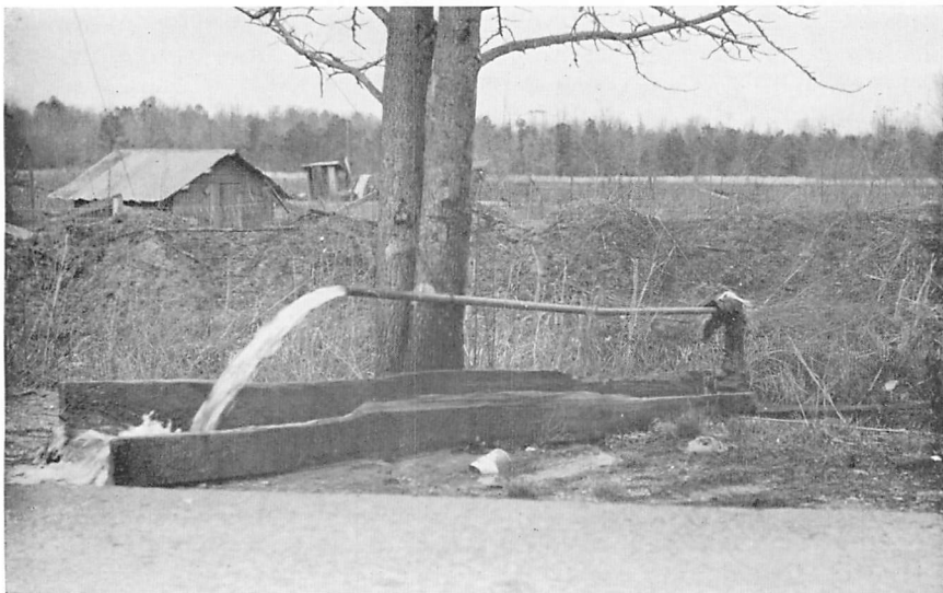
Figure 3.—Artesian well flowing continuously in Itawamba County. Depth, 140 feet in sand and gravel of Tuscaloosa group; rate of flow, about 50 gpm; temperature of water, 62° F.
