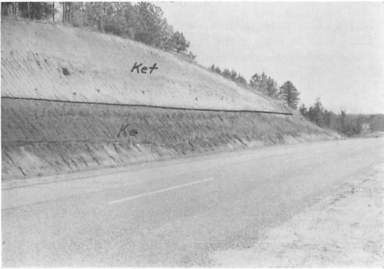
Figure 10.—Contact between lower Eutaw (Ke) and Tombigbee sand member (Ket) in cut on State Highway 30 at the Prentiss-Tishomingo County line. (SE.¼, Sec.5, T.5 S., R.9 E.). February, 1959.
