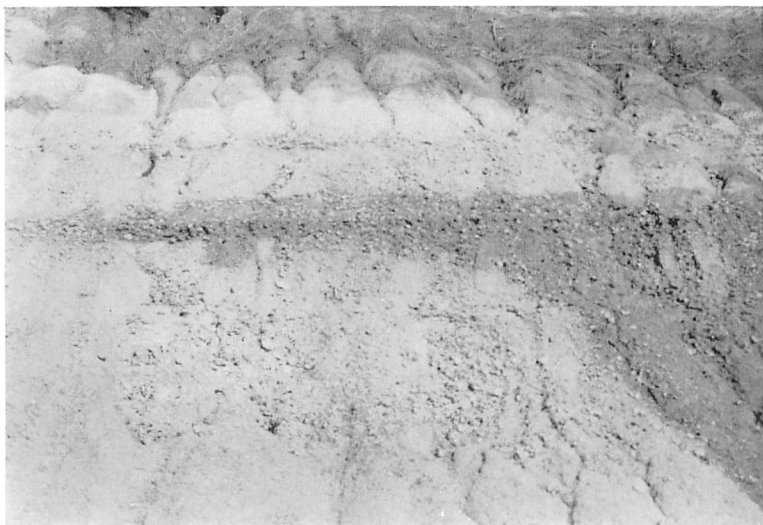
Figure 17.—Shell beds in chalk of the Demopolis exposed in cut of State Highway 370 on Northeast facing valley wall of Okolalah (SW. \frac{1}{4} , SE. \frac{1}{4} , Sec. 33, T. 6 S., R. 6 E.). February, 1959.
