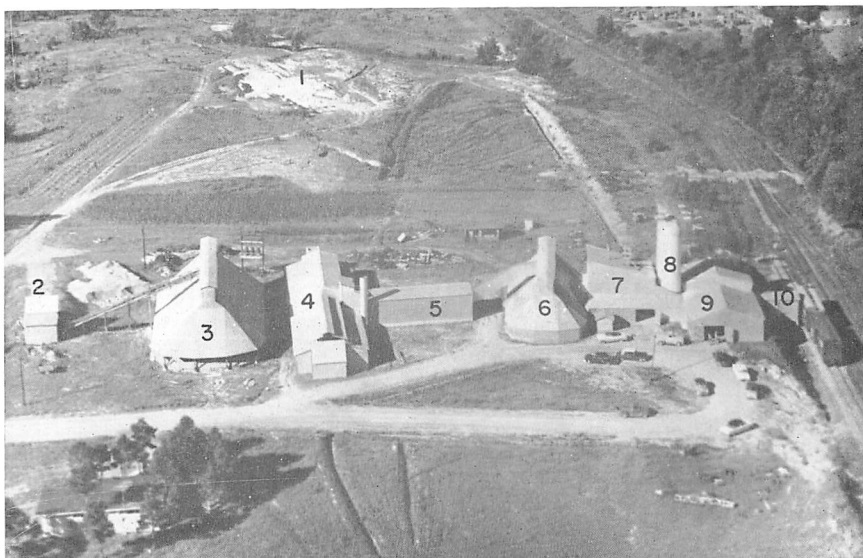
Figure 22.—Plant of Howell-Southern Products, Inc., Ripley, Tippah County, Mississippi, which produces fired clay aggregated for absorbent and deodorizing purposes: (1) clay pit—basal Porters Creek, (2) shredding shed, (3) dry shed, (4) kiln building, (5) cooler, (6) product storage, (7) screening and crushing, (8) silos, (9) bagging, and (10) loading. Photo by Richard Allin, December, 1958.
