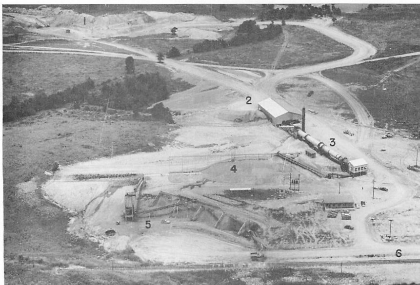
Figure 24.—Miss-Lite aggregate plant of Jackson Ready-Mix Concrete at Cynthia, Hinds County, Mississippi: (1) pits opened in the Yazoo clay, (2) clay dry shed, (3) rotary kiln, (4) clinker storage area, (5) grinding, screening and storage of graded aggregates, and rail or truck shipping facilities. Photo by Frank Noone, July 2, 1958.
