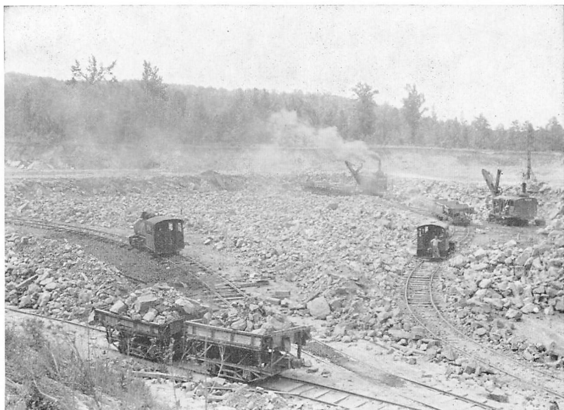
Figure 29.—Asphaltic oolitic limestone of Chester age, produced by Alabama Asphaltic Limestone Company as a natural rock asphalt paving material, south of Margerum, Colbert County, Alabama, (NE. \frac{1}{4} , Sec. 12, T.4 S., R. 15 W.), 3- \frac{1}{2} miles east of Tishomingo County line. May 26, 1941.
