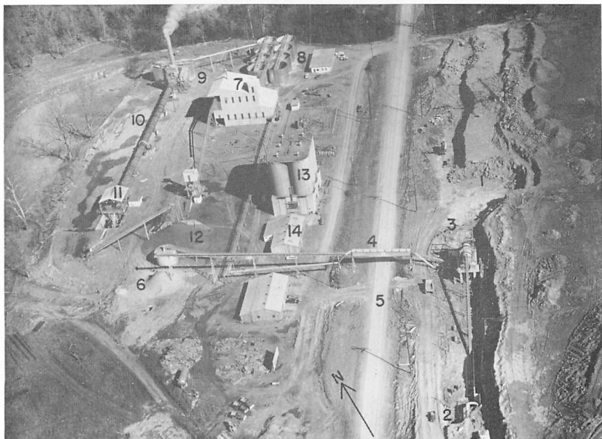
Figure 32.—Mississippi Valley Portland Cement Company plant at Haynes Bluff, Warren County, Mississippi: (1) quarry face, (2) primary crusher, (3) washing and screening, (4) overhead conveyor, (5) Mississippi State Highway 3, (6) limestone storage, (7) milling house, (8) slurry blending and storage, (9) slurry tanks and kiln feeding equipment, (10) kiln, (11) clinker cooler, (12) clinker storage, (13) silos, and (14) sack house. Photo by Newton Advertising Agency, January 25, 1959.
