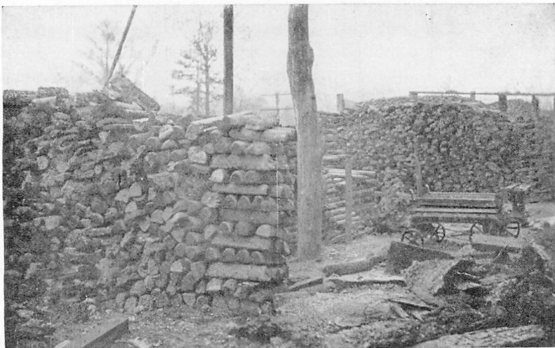
Figure 42.—Pig iron (125 tons) smelted by the furnace at Winborn. (M. G. S. Bull. 12, Fig. 13) (M. G. S. Bull. 80, Fig. 28).
