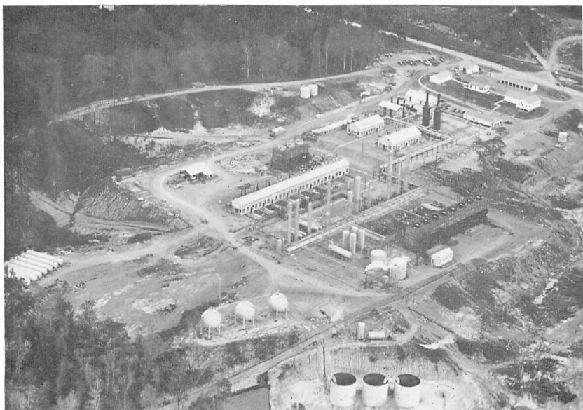
Figure 11.—The California Company's Cranfield Field Unit, Adams County, Mississippi, showing U. S. Highway 84 (right background), field offices, unit cycling plant and a few individual lease installations. The plant is designed to conserve reservoir energy in the primary recovery of Tuscaloosa oil, to recover the liquid hydrocarbons produced with the gas from the Tuscaloosa gas cap, and to return the stripped gas to the reservoir. Photo by Elwood M. Payne, October 24, 1947.
