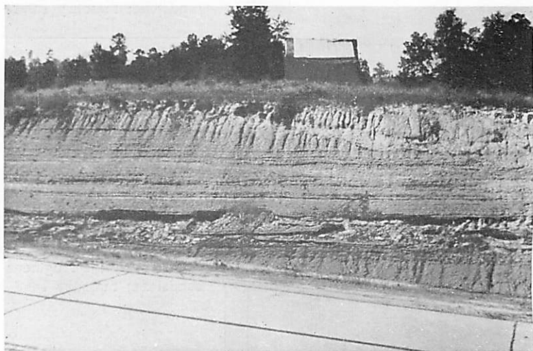
Figure 3.—Interbedded sand and shale in upper member of Fearn Springs formation. Highway cut on U. S. 45, 0.5 mile north of the Lauderdale-Kemper County line. V. M. Foster, Photo. October 10, 1938. (M. S. G. S., Bull. 41, Fig. 7).
