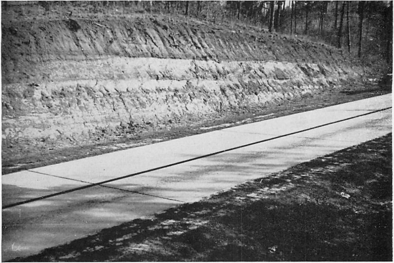
Figure 18. —Weak concretionary sandstone development in weathered exposure of the Potterchitto member. Cut on Highway U. S. 11, 1.2 miles north of railroad overpass near Wautubbee Station, Clarke County.
