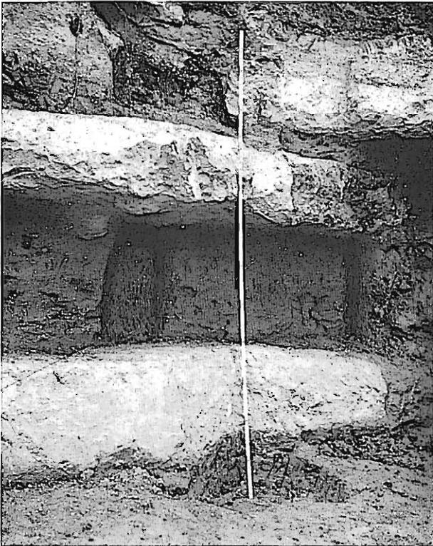
Figure 8.—Glendon limestones and marls in a close-up view of Test E 10, showing relationship of limestones and marls and method of sampling. February 21, 1939.
