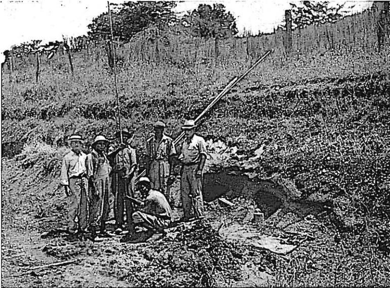
**Figure 12.**—“Coming out” of test hole E 161, one fourth mile south of Yokena; elevation 108 feet; drilled to top of Glendon limestone at 168 feet. July 28, 1939.
