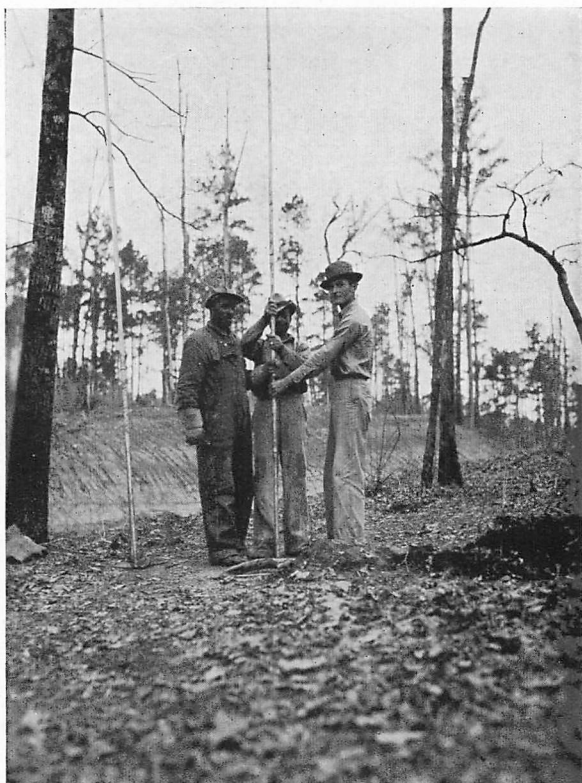
Figure 24.—Removing auger from the 76-foot test hole 57 on the property of Melvin McCully (NW. \frac{1}{4} , SE. \frac{1}{4} , Sec. 15, T.15 N., R.12 E.). The efficiency of boring wells with this type equipment has not been exhausted at this depth.---March 10, 1938.
