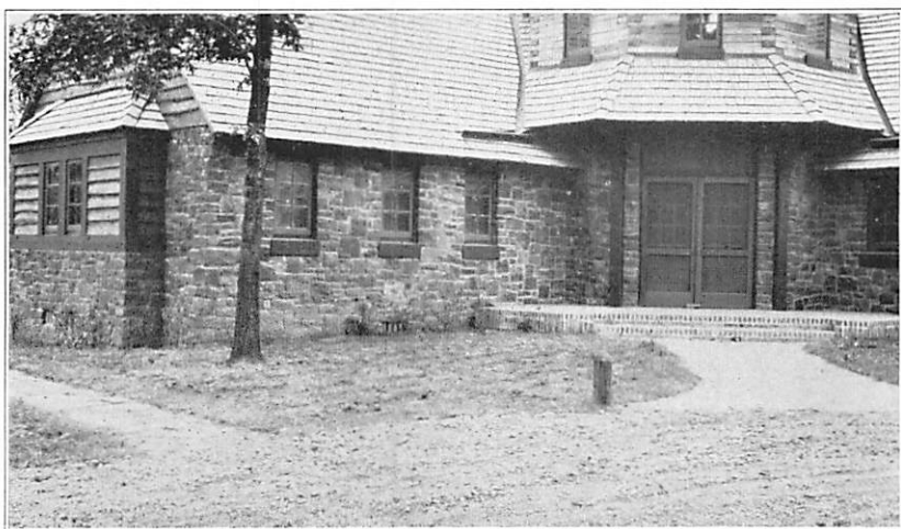
Figure 7. —Detailed construction of the Lodge in Tombigbee State Park. The lumber came from the trees that were cleared for the lake bed; the dark ferruginous sandstone blocks, from Pontotoc and Itawamba counties; the light colored sandstone, from the Highland Church sandstone of the Forest Grove formation at Bay Springs, Tishomingo County.---Photographed June 5, 1936.
