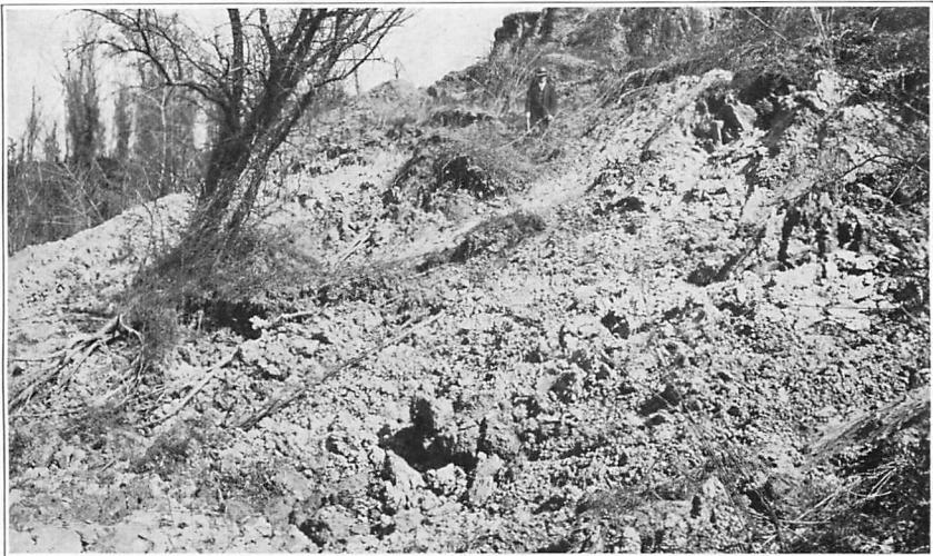
Figure 1.—Landslide during the winter of 1934-35 near the line of the proposed highway at the end of the second spur ridge, B Plate 1, east of the Yazoo River at Yazoo City. It embraces practically all the material from the clay contact to the top of the Loess.
