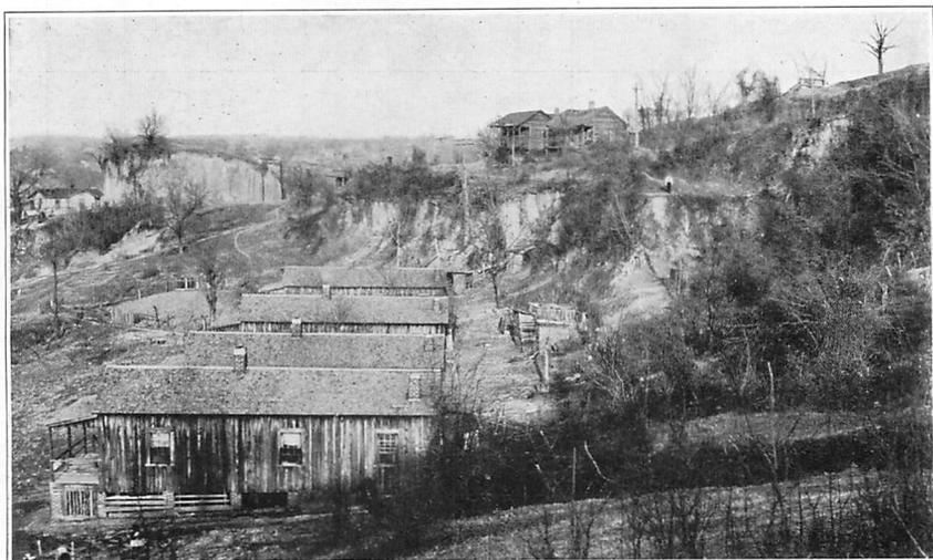
Figure 8.—Looking east toward the proposed line of the highway leading up the east bluff of the Yazoo Valley. The escarpments and terraces of the landslides are so masked by age as to be readily mistaken for peculiar loess erosion features; an example showing the necessity for inspection by a trained and experienced geologist.
