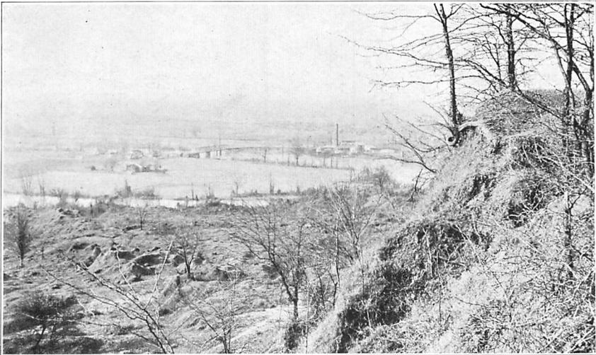
Figure 7.—Landslide topography embracing practically the whole vertical face of the east bluff of the Yazoo Valley at this point --west side of the first spur ridge, A Plate 1, east of the river. The camera, trained North 22° West toward the proposed bridge site, shows the area south of the site and almost but not entirely to the banks of the river.
