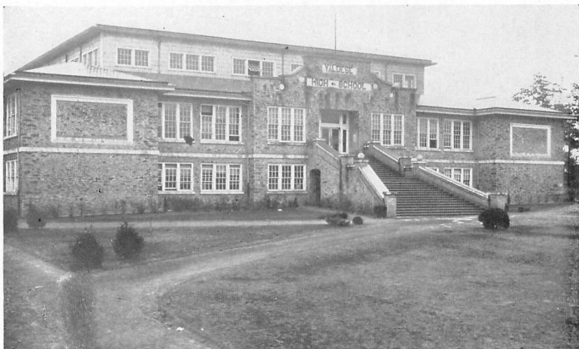
Figure 8.—Valdese High School, built of flat field stone at Valdese, North Carolina, by immigrants from the Franco-Italian Alps.
