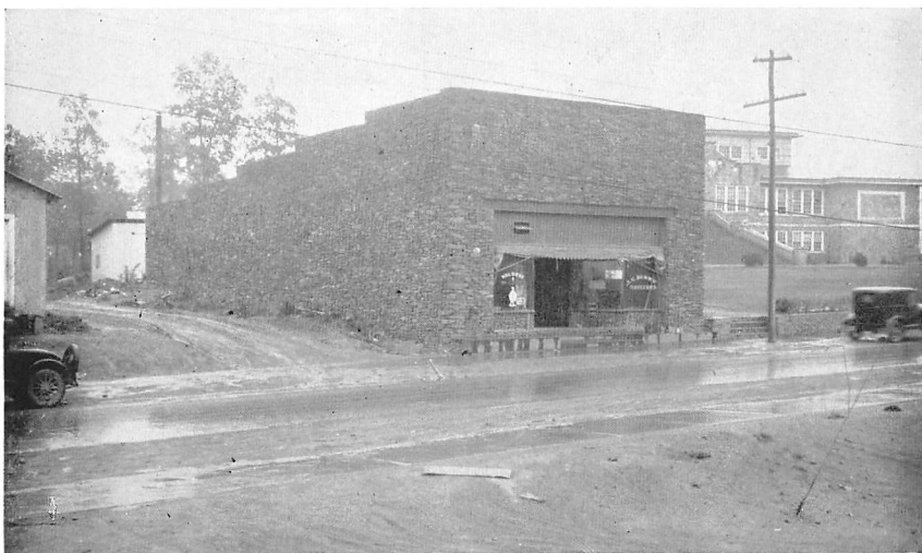
Figure 9.—A business room, safe, solid, substantial, satisfying—built of flat field stone at Valdese, North Carolina, by sons of the Franco-Italian Alps.
