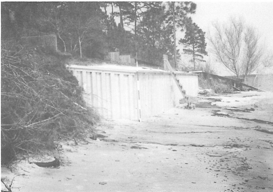
Figure 11. Isolated bulkhead, Central Belle Fontaine. (scale is in feet)
