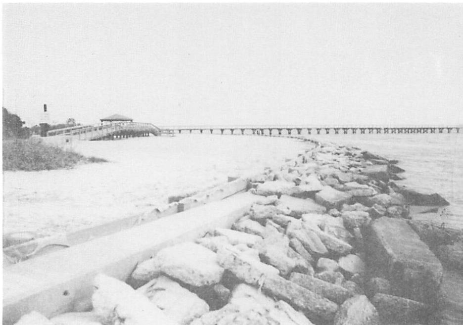
Figure 16. Park and pier area protected by riprap in the Pointe aux Chênes area.
