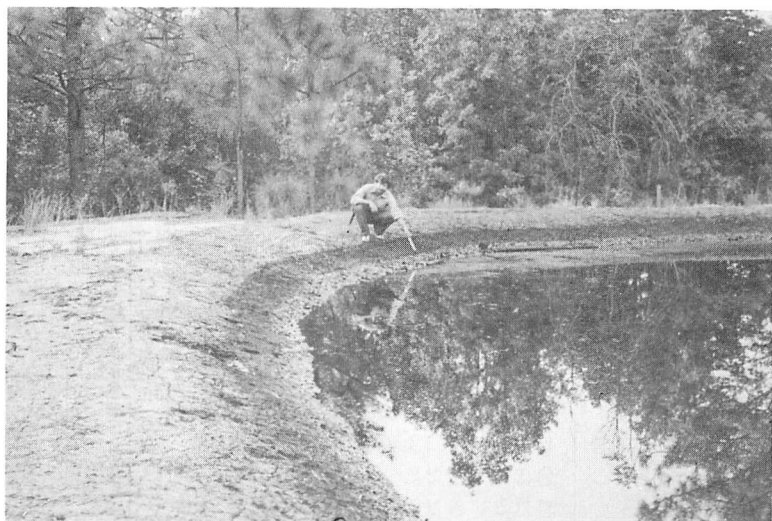
Figure 7.—Salt-water evaporation pit that has a high seepage rate. The knife point is at the fluid level of the pit approximately three hours prior to this photograph. Location is in Eucutta Oil Field, in NW/4, SE/4, SE/4, Sec. 12, T.9N., R.9W. August 1973.
