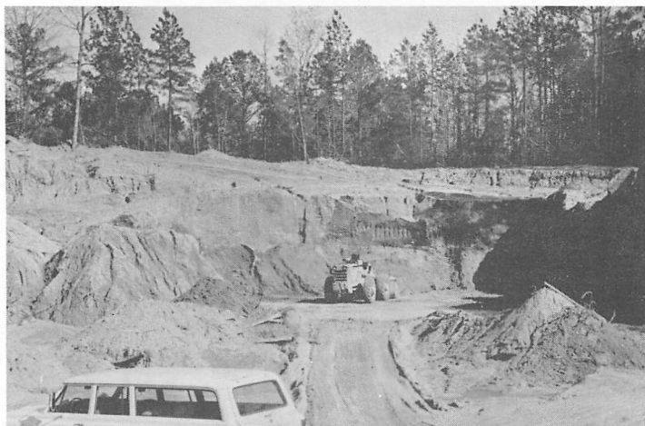
Figure 22.—Excavating gravel of Citronelle age with front-end loader for use on county roads.
